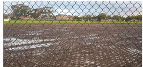
**NEW INFIELD:** The excavations works have been done and the crushed rock has been put down.
